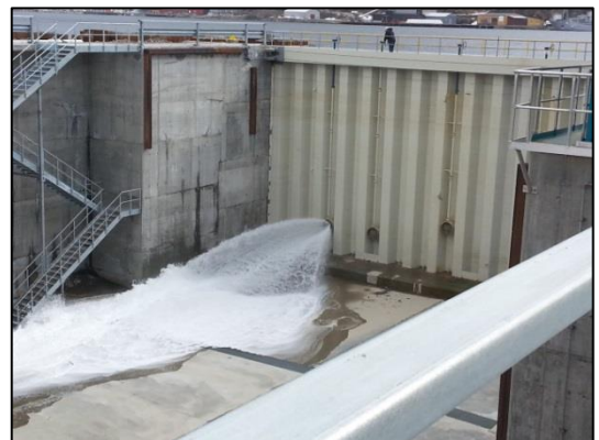
HAMEK'S new dry dock (145 x 27 x 9,5 meters)
